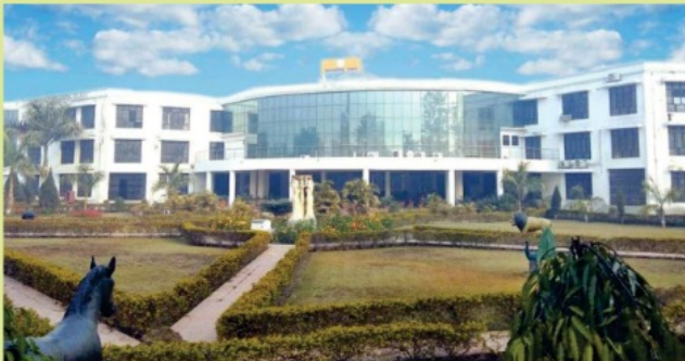
Administrative Building ANDUA&T, AYODHYA
