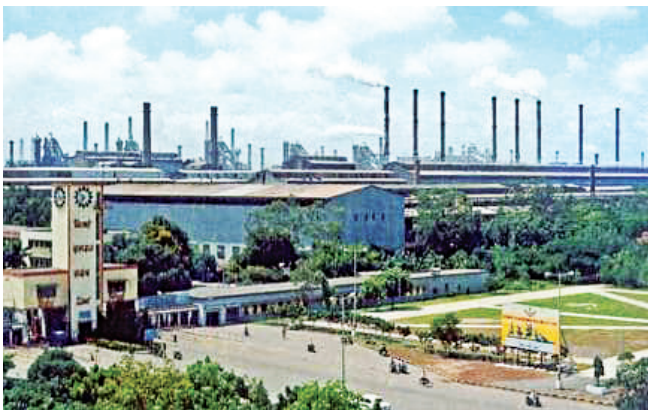
Bhilai Steel Plant
