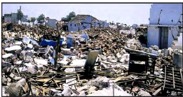
Figure 5.2 :The Bhuj earthquake 26 th January,2001
