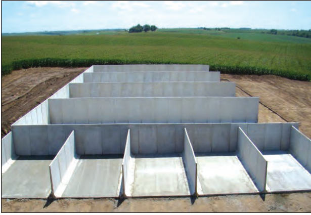
Fig. 8.5 Horizontal trench silo
